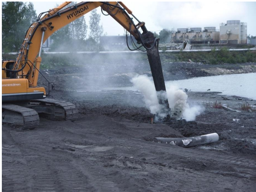
Stabilization work ongoing in Sampaanala Bay
