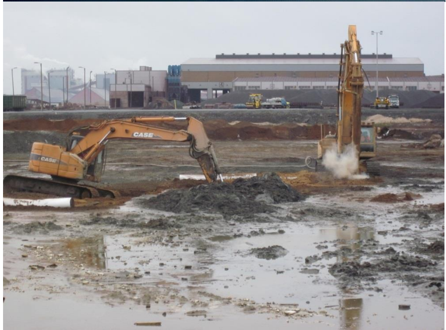
Ongoing mass stabilization
