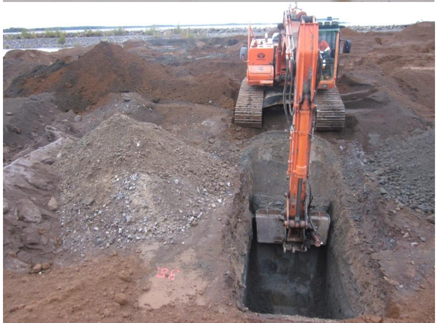
Test pit for technical quality control
