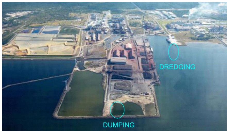
Dredging and dumping areas
