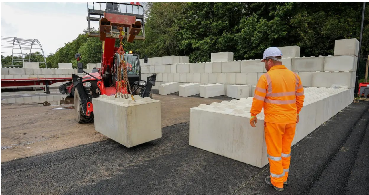
Figure 3.2. Installation of PICBs with reacher stacker. (Poundfield Precast, 2023).
