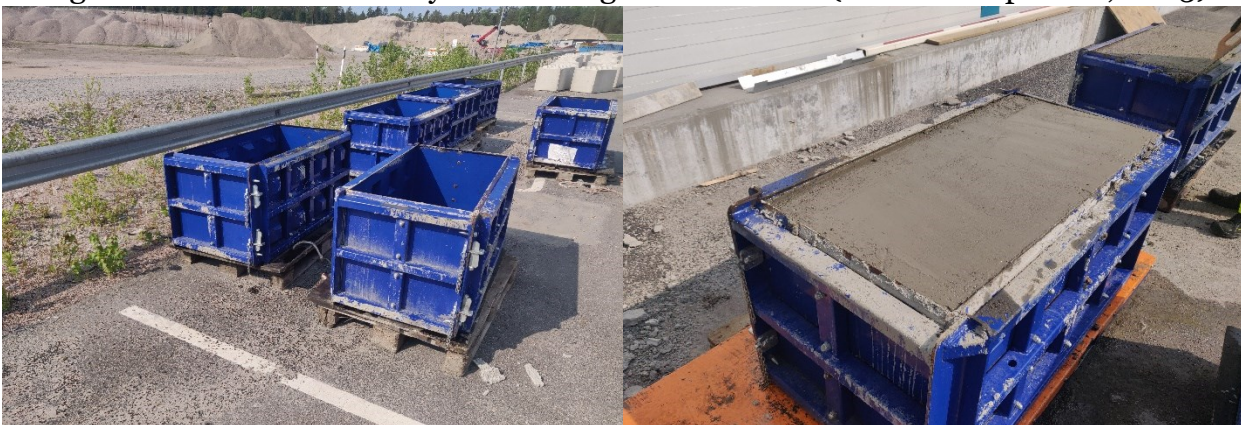
Figure 3.3. Reusable formwork for PICB in HSY Ämmässuo.
