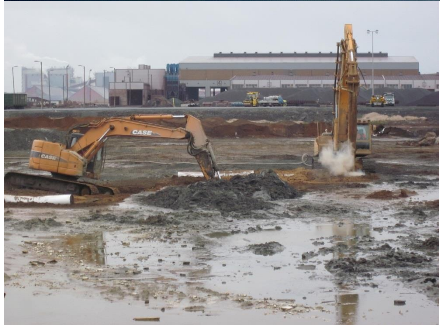
Ongoing mass stabilization
