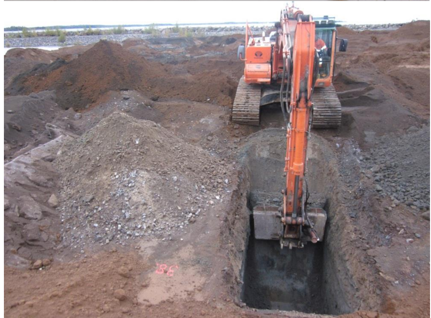
Test pit for technical quality control
