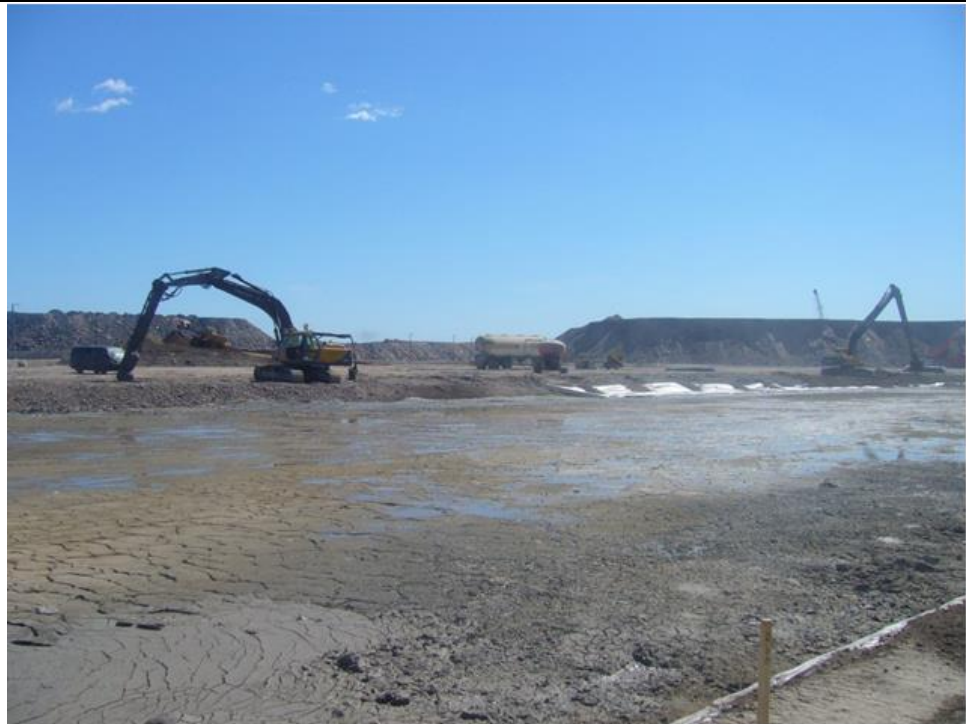
Stabilization works in progress.
