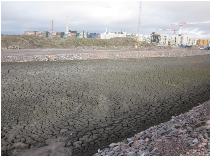
Stabilized sediments temporarily stored in stabilization basins in Jätkäsaari
