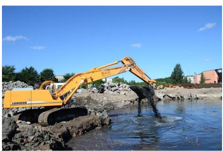
Stabilization of the surplus soft clay placed in the pit. In the back, a loading embankment is constructed. This functions as a working platform for the stabilization equipment. It also allows for the compaction of the stabilized soil layer during the curing time.
